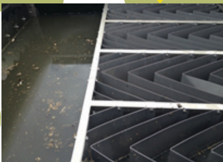
The cross-flow lamella settler
