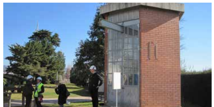
DESSIN's well at the Llobregat Demo Site.
