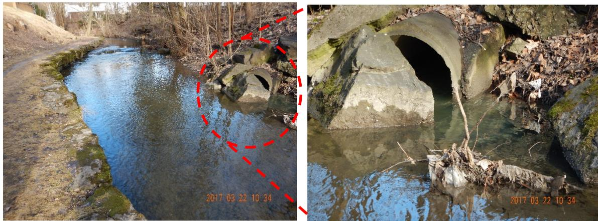
Figure 17: Photo taken at OPAK by the research team. Right hand picture shows litter at the outlet of a discharge pipe, believed to be from the CSO HO62.
