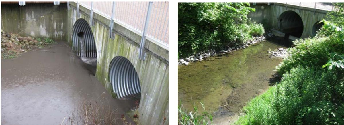
Figure 16: Hoffselvpromenaden/Glippen. Left: Overflow, 06.04-2016. Right: Normal conditions, 01-06-2017.
