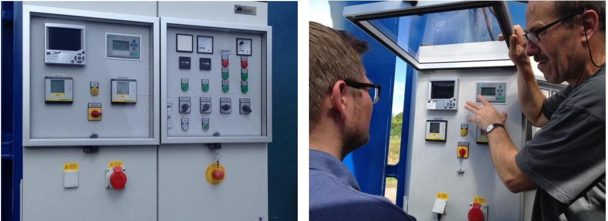
Figure 22 Electric cabinet for automated container control.
