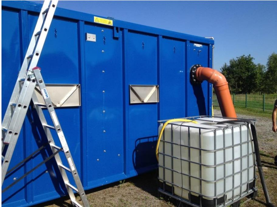
Figure 20 Installation of a fresh water tank feeding the container's self-cleaning mechanism after every container operation.
