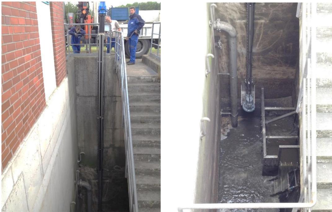
Figure 11 Installation of the pump in the CSO pump sump.
