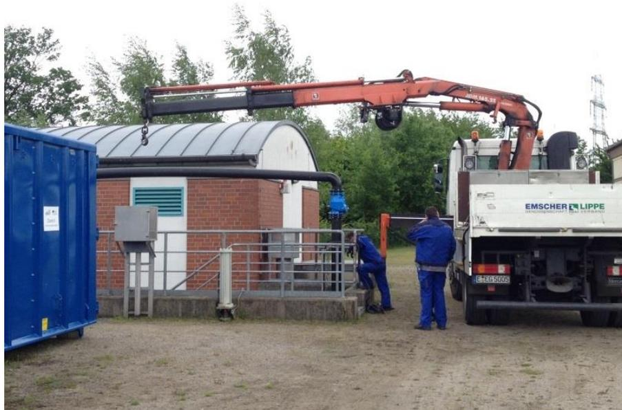
Figure 13 Installation of the inflow pipe from the pump to the container.
