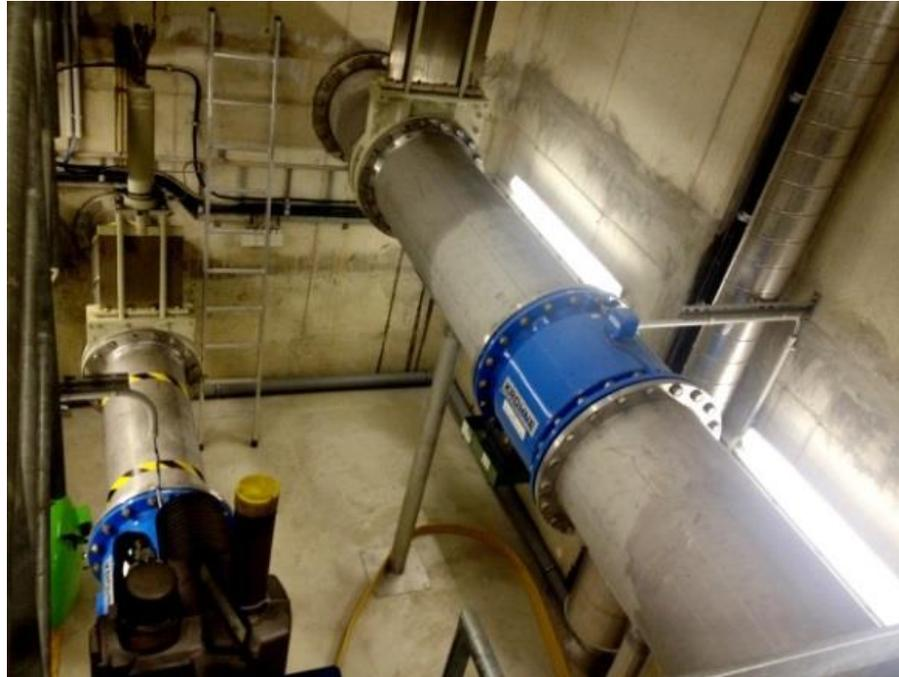
Figure 73 Newly installed second throttle at CSO Strickerstr.
