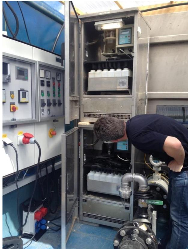
Figure 27 Installation of automatic sampler in the electric cabinet.
