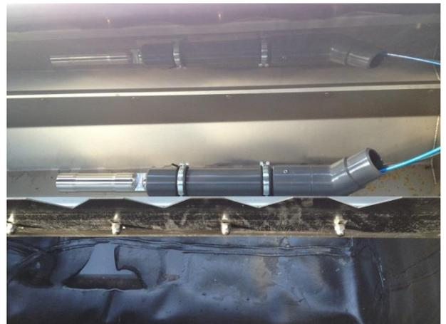
Figure 26 Installation of s::can probes at in- and overflow.
