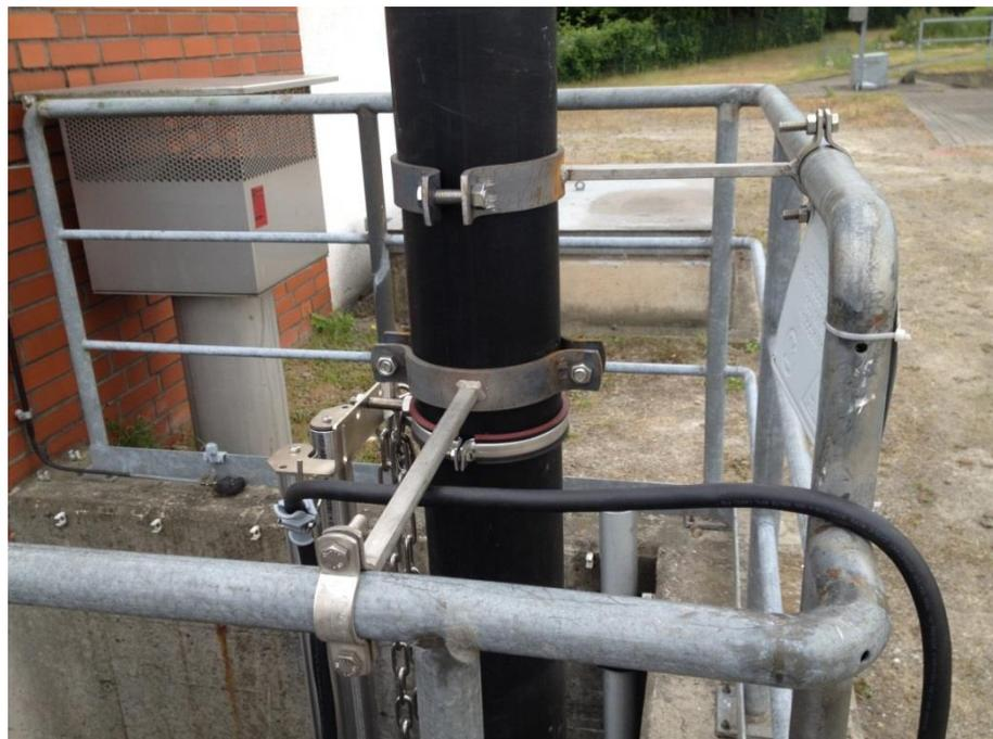
Figure 15 Required reinforcement of the attachment of the inflow pipe.
