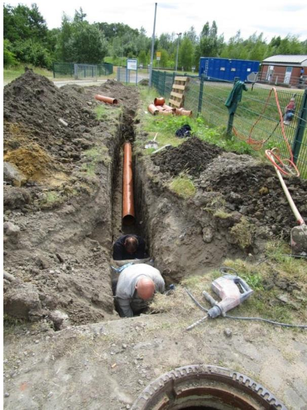
Figure 17 Construction works of the underground discharge pipe directing the treated water to the next sewer.
