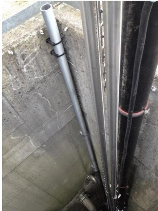
Figure 12 Installation of the protection pipe for the pump's level sensor.
