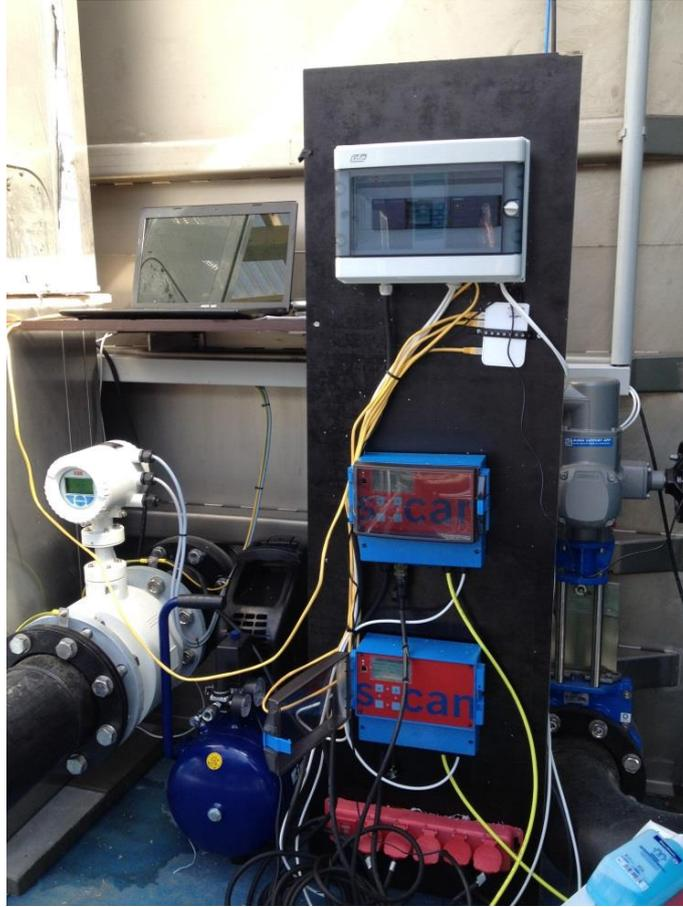
Figure 25 Installation of s::can control unit in the electric cabinet.
