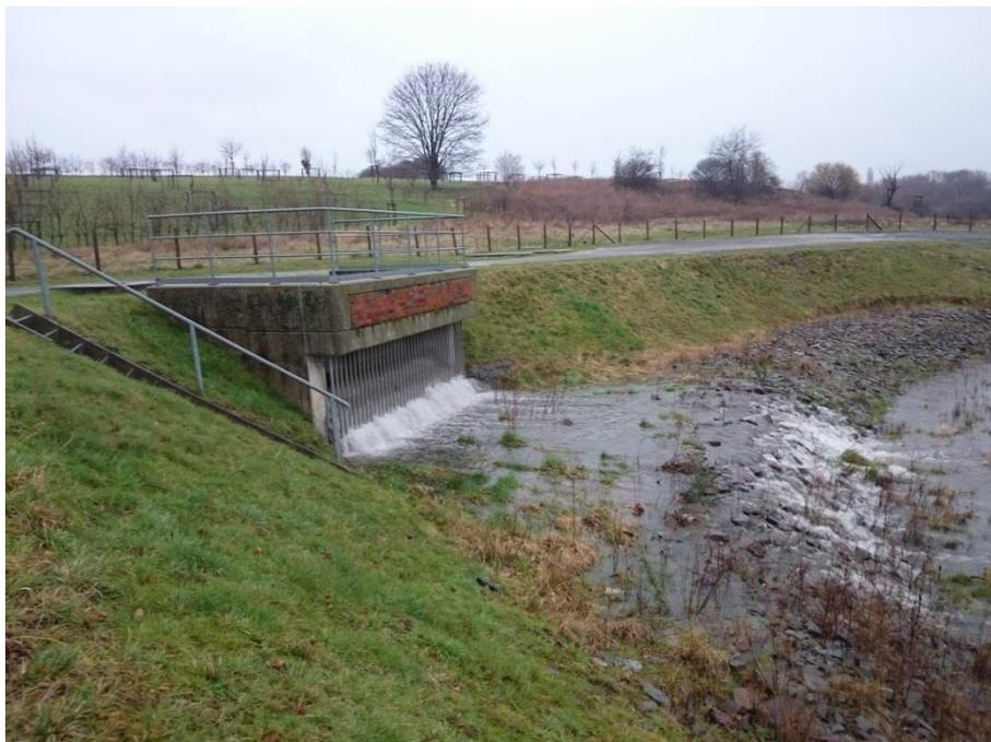
Figure 1 Combined sewer overflow discharging combined sewage into a nearby receiving stream.
