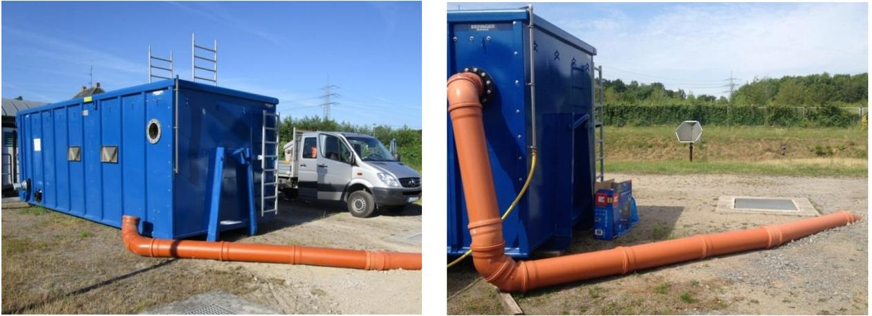
Figure 16 Attachment of the discharge pipe to the container, discharging into the next sewer.
