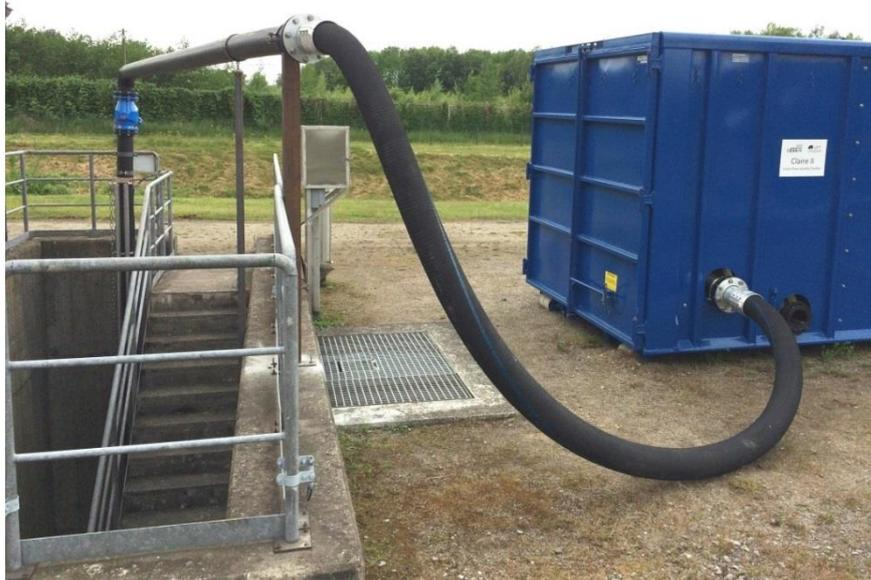
Figure 14 Installed inflow pipe and hose from the pump to the container.
